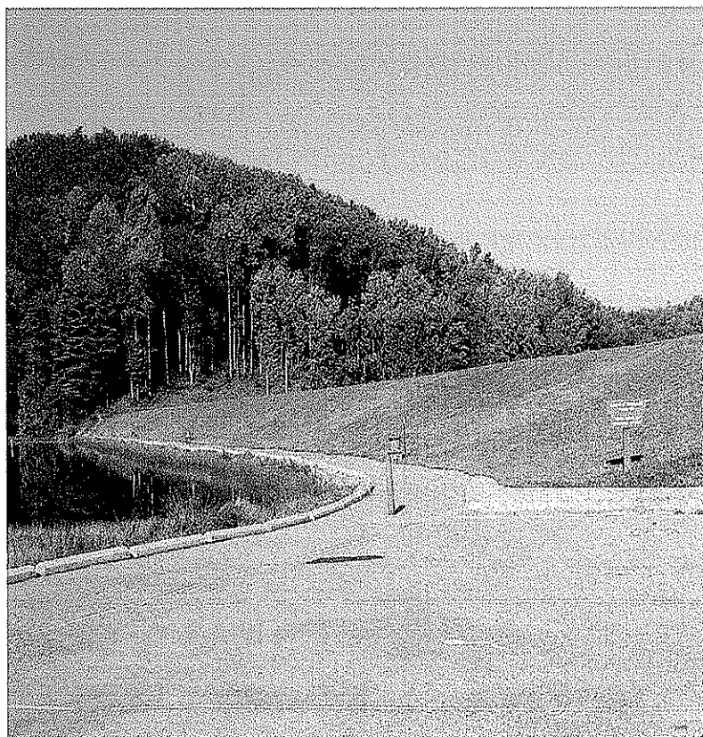
TETER CREEK DAM MODIFICATION, BARBOUR CO., WV
