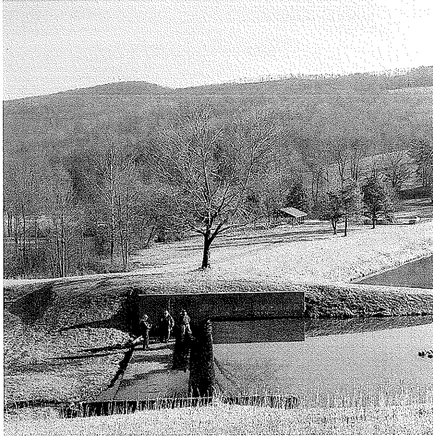
BELINGTON DAM MODIFICATION, BELINGTON, WV
