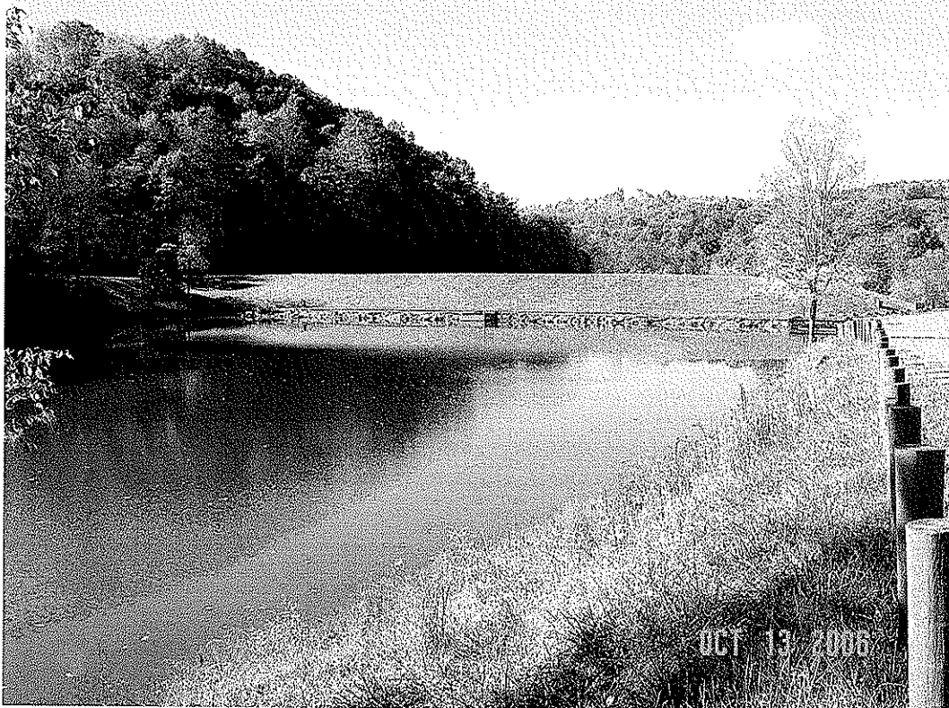
JIMMY LEWIS DAM MODIFICATION, MERCER CO., WV
