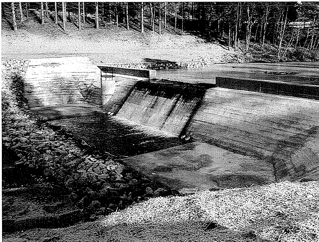
THOMAS DAM MODIFICATION, THOMAS, WV
