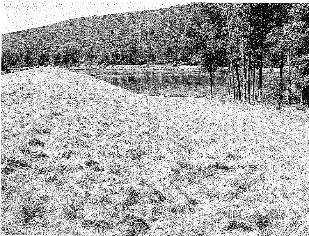
WARDEN LAKE DAM MODIFICATION, HARDY CO., WV
