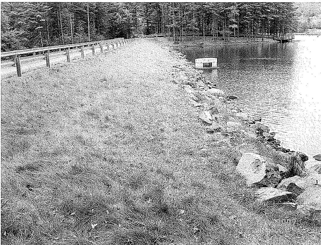
MONCOVE DAM MODIFICATION, MONROE CO., WV
