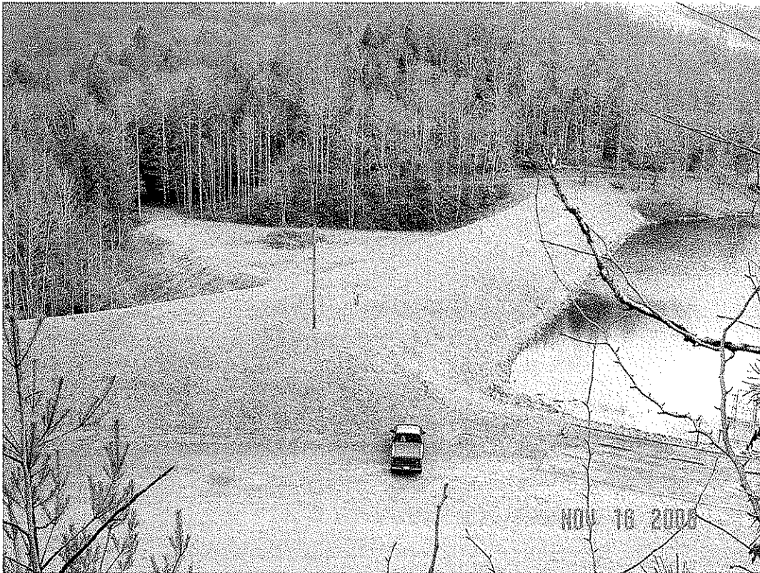
PLUM ORCHARD DAM MODIFICATION, FAYETTE CO., WV
