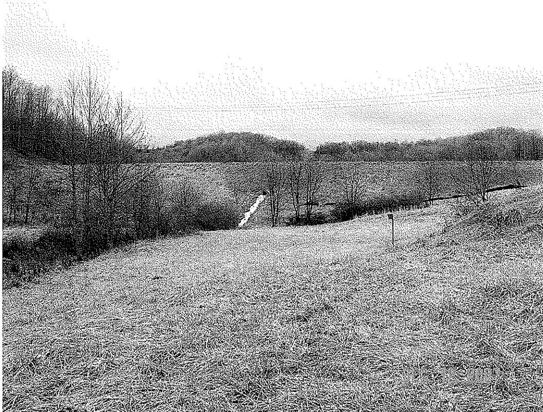
LEMLEY DAM MODIFICATION, MONONGALIA CO., WV
