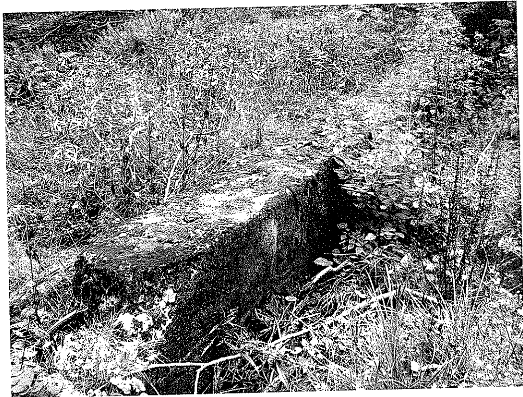
Picture 3 is an on-site foundation located in a small stream.
