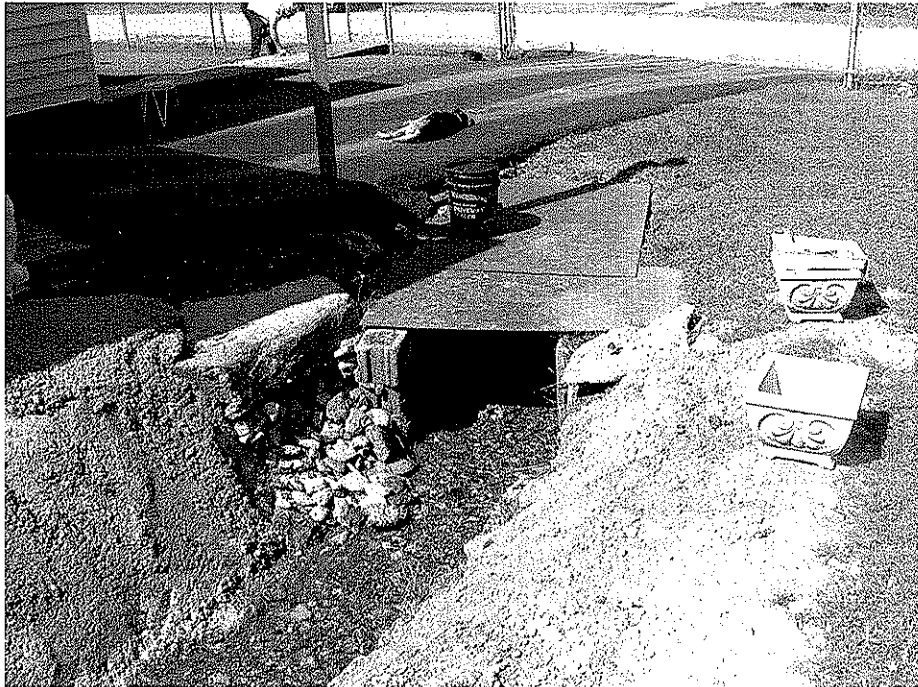
Picture 5 shows the pipe culvert inlet.
