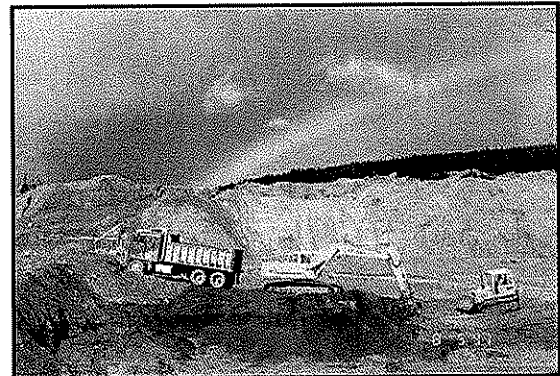
Removal of tailing from floodplain
