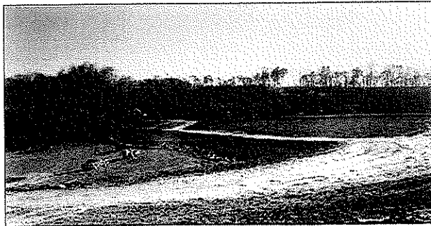
Construction of the cap system was completed in phases. A buttress was constructed over the face of the landfill to flatten slopes to 4 horizontal to 1 vertical to improve stability of the cap.
