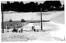
The leachate collection piping system consists of 8" HDPE perforated pipes placed in the stone trenches. Two 30,000-gallon fiberglass-reinforced, double-wall, underground storage tanks were proposed for both cells. Motor operate d plug valves were designed for leachate outlet piping to control influent flow to the tanks. The EPA HELP Model was used to estimate leachate generation.
