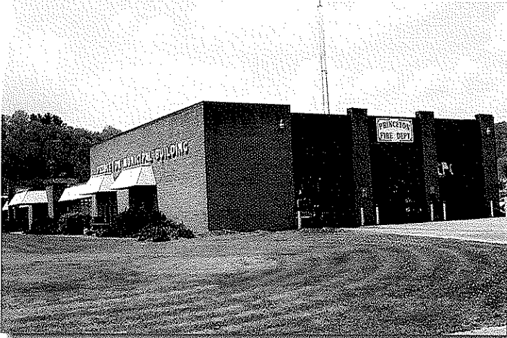
Princeton Municipal Building & Fire Department
