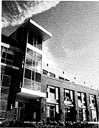
WVU Transportation Center & Garage
