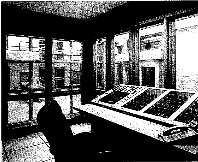
Control Room at Housing Units
