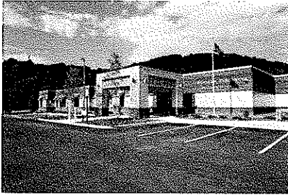
Western Virginia Regional Jail
