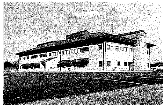
WVDOH D-10 Office Building, Gardner, WV
