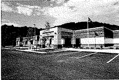
Western Virginia Regional Jail
