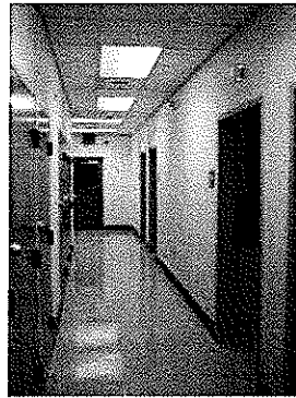
Completed corridor with line of sight to exam rooms
