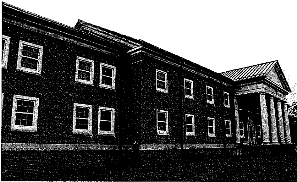
Jones Building Renovations Industrial, WV
