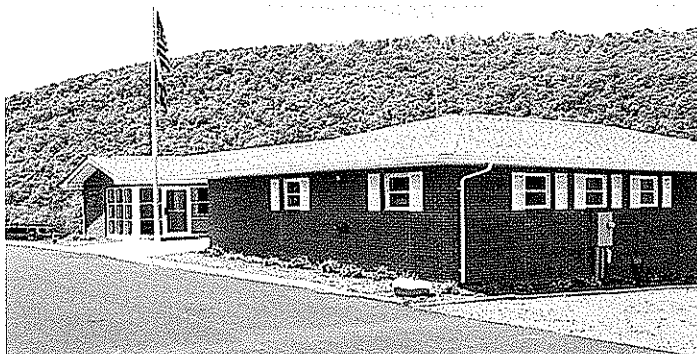
Architectural and Engineering design for new addition and renovations to the detachment in Pendleton. Included in the structure are the following departments: DMV, BCI, 911, & regular squad space.
