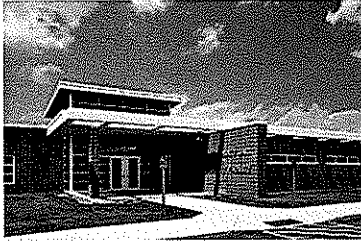
*ALLEGANY COUNTY JAIL AND PUBLIC SAFETY FACILITY AMITY, NY
