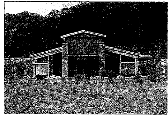
Sandstone Visitor/Orientation Center. The project site is located in a remote section of West Virginia, with few public utilities available as energy sources for the project
