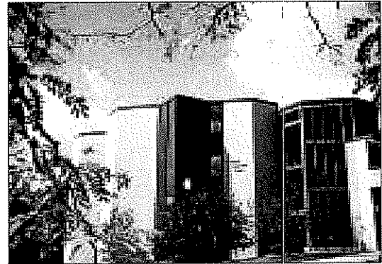
Fairmont State College. H.F. Lenz Company upgraded the electrical distribution system for Hunt Haught Hall.
