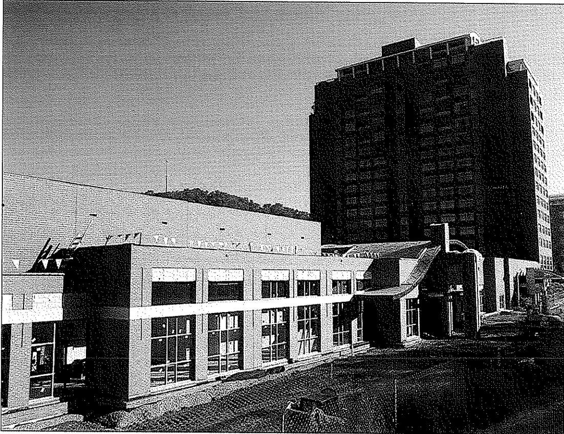
(Currently Under Construction)
