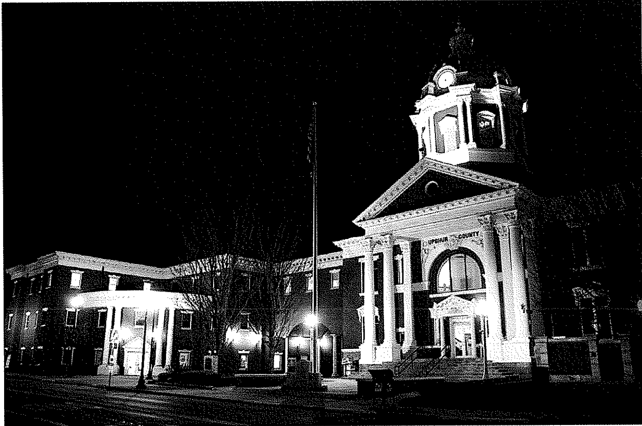
Upshur County Courthouse Complex
