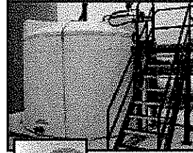
Double-Wall Containment "Tank within a Tank"
