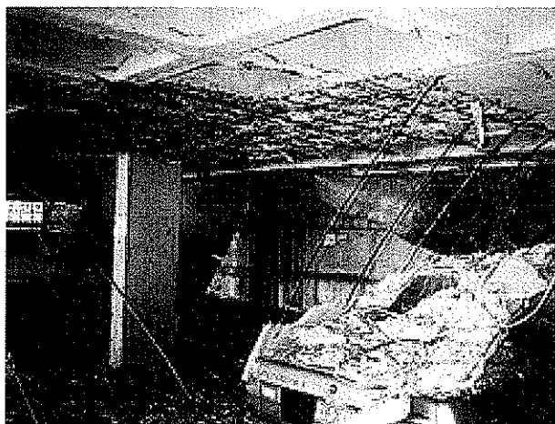
Damage from chloride-based deicers
