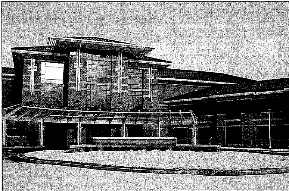
WV Veterans 120 Bed Nursing Facility Clarksburg, WV
