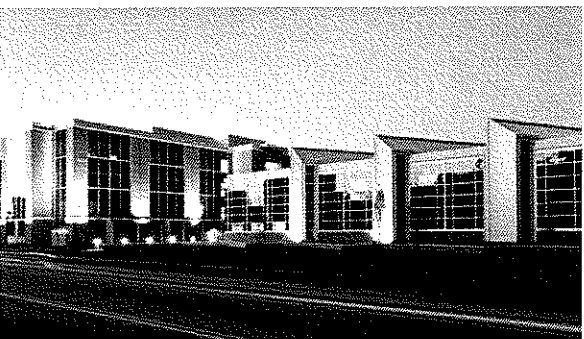
International Brotherhood of Electrical Workers Local #5 Headquarters
