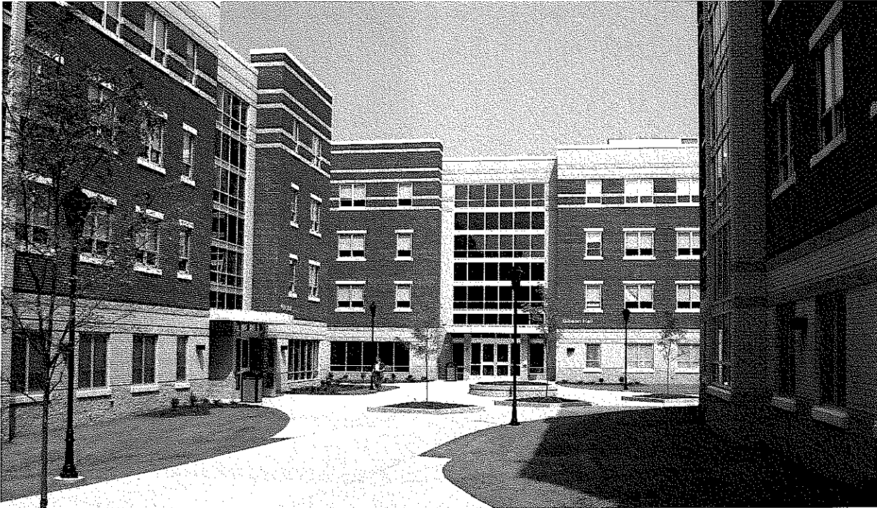
Marshall University Student Housing Complex
