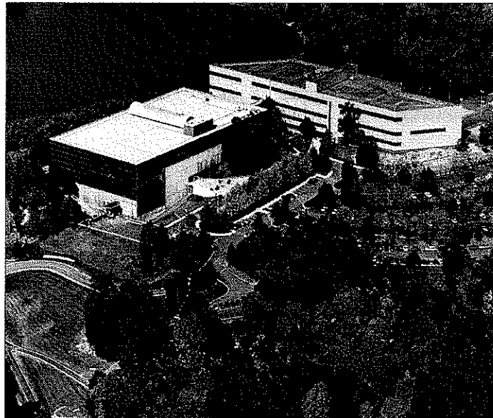
Above: the Sterling Forest, NY Enterprise Recovery Site has over 200,000 square feet of raised floor
