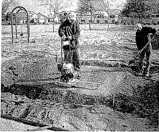
Start with a base of compacted aggregate
