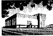
Corporate Headquarters Facility Blue Cross / Blue Shield of West Virginia Charleston, West Virginia
