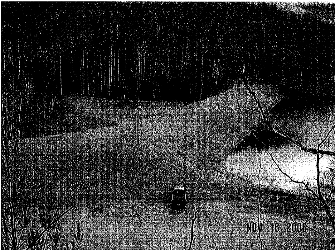
PLUM ORCHARD DAM MODIFICATION, FAYETTE CO., WV
