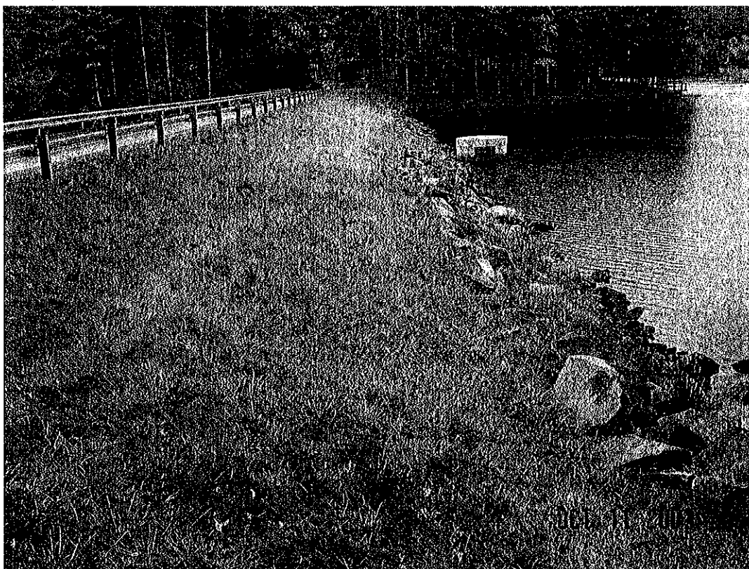
MONCOVE DAM MODIFICATION, MONROE CO., WV
