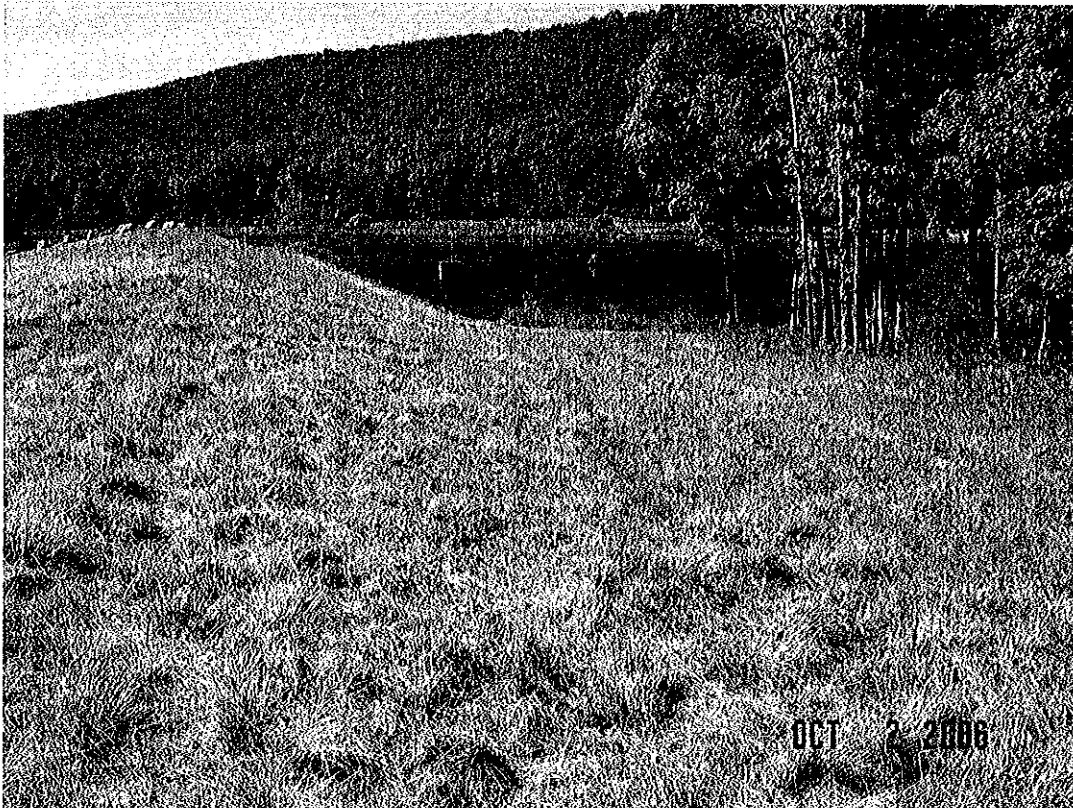
WARDEN LAKE DAM MODIFICATION, HARDY CO., WV
