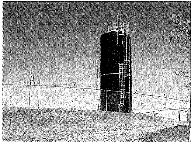
43,000 Gallon Salem Ridge Water Storage Tank
