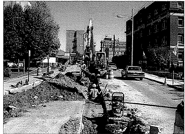
Completed in 2003 Main Street Waterline Replacement Project New 12" Ductile Iron Pipe Installation
