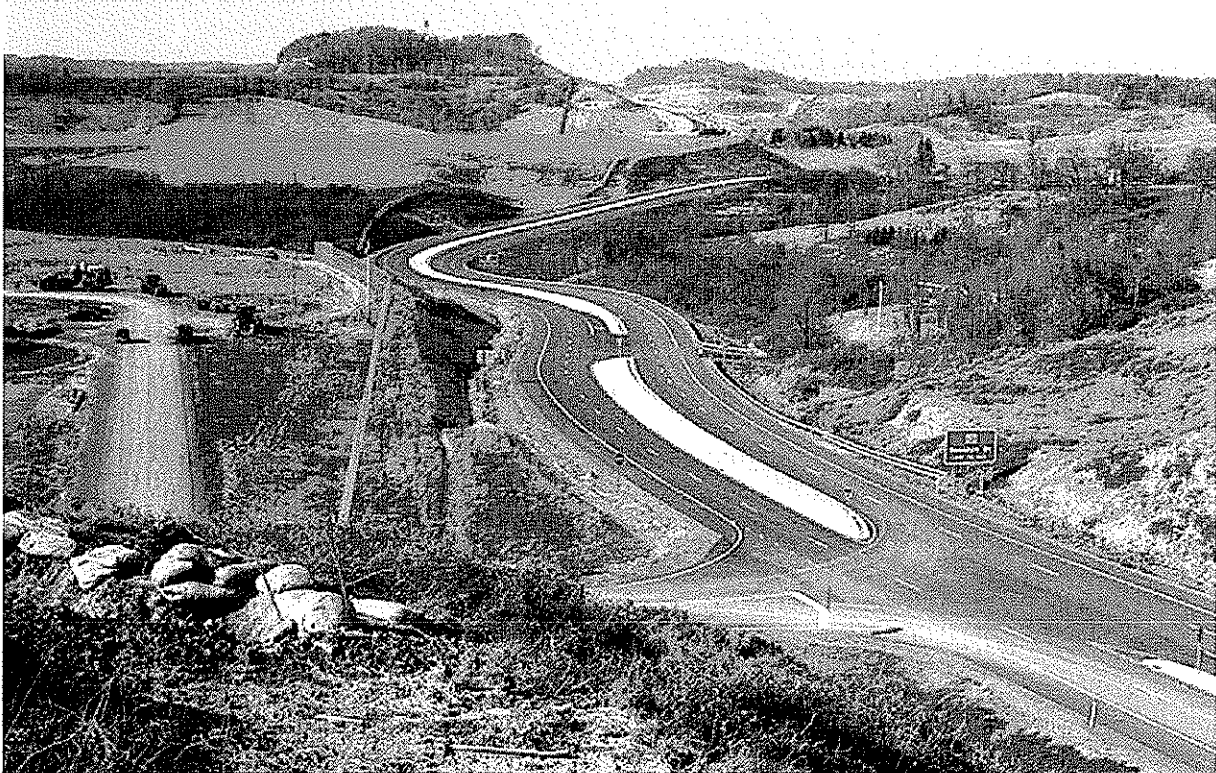
ROUTE 279, NORTH BRIDGEPORT BYPASS - COMPLETED IN 2000
