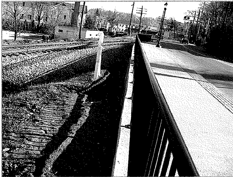
Safety Rail Along North Side of Main Street
