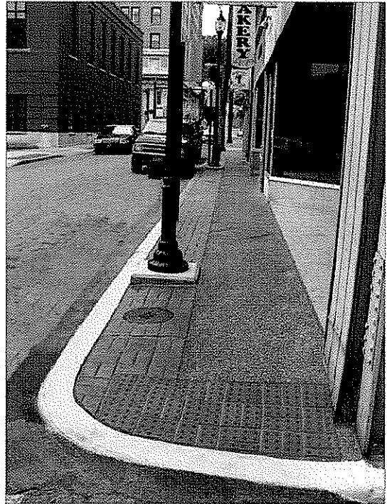
West Side of South Third Street
