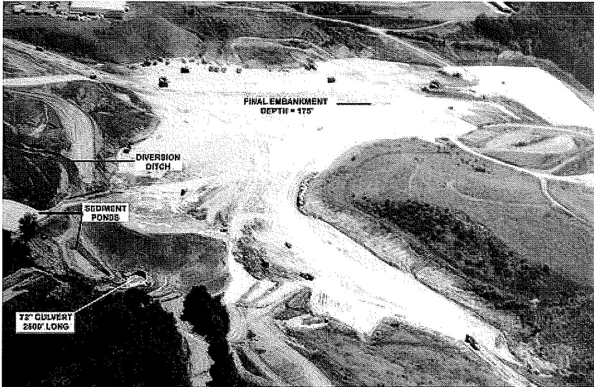
BENEDUM AIRPORT RUNWAY EXTENSION PROJECT - 1999
