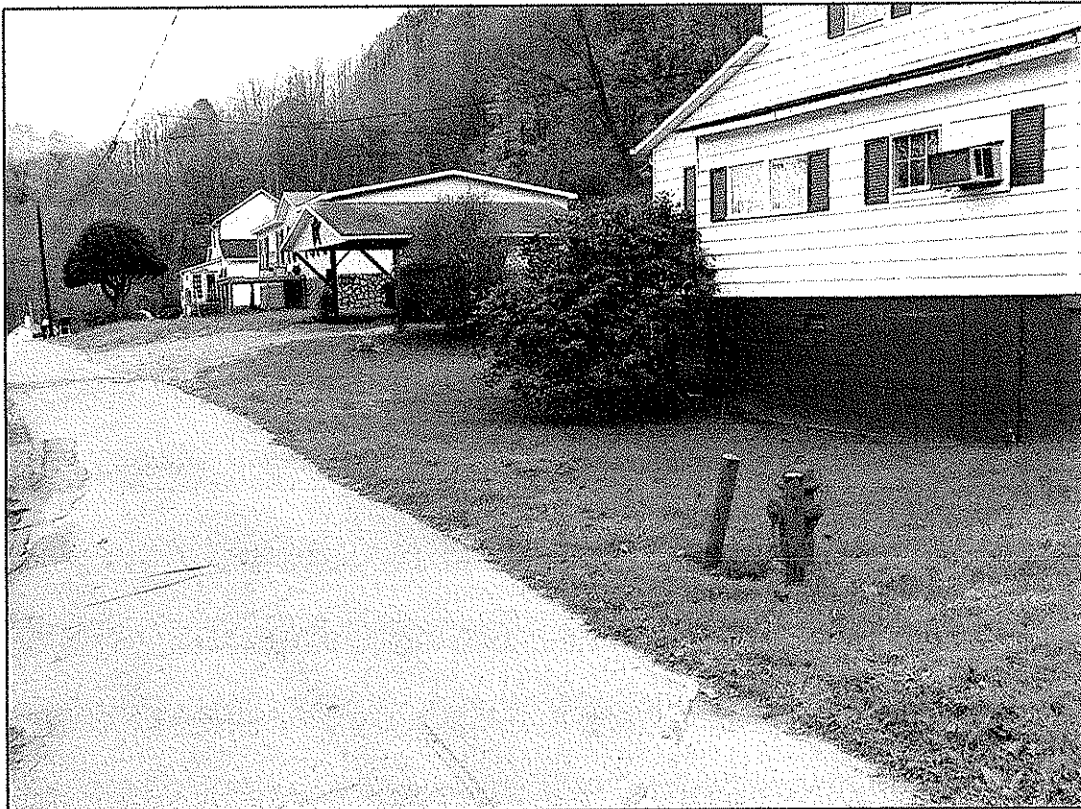
PHOTO 2 – AREA OF PONDING WATER DURING WET WEATHER
