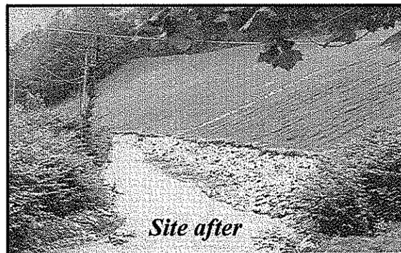
all vegetation on the refuse pile, thorough extinguishing of all burning refuse, regrading and revegetation of refuse to stable slope, demolition of tippie, and sealing of three portals.
