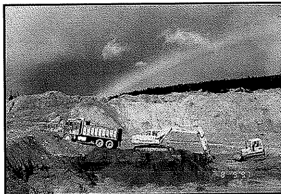
Removal of tailing from floodplain
