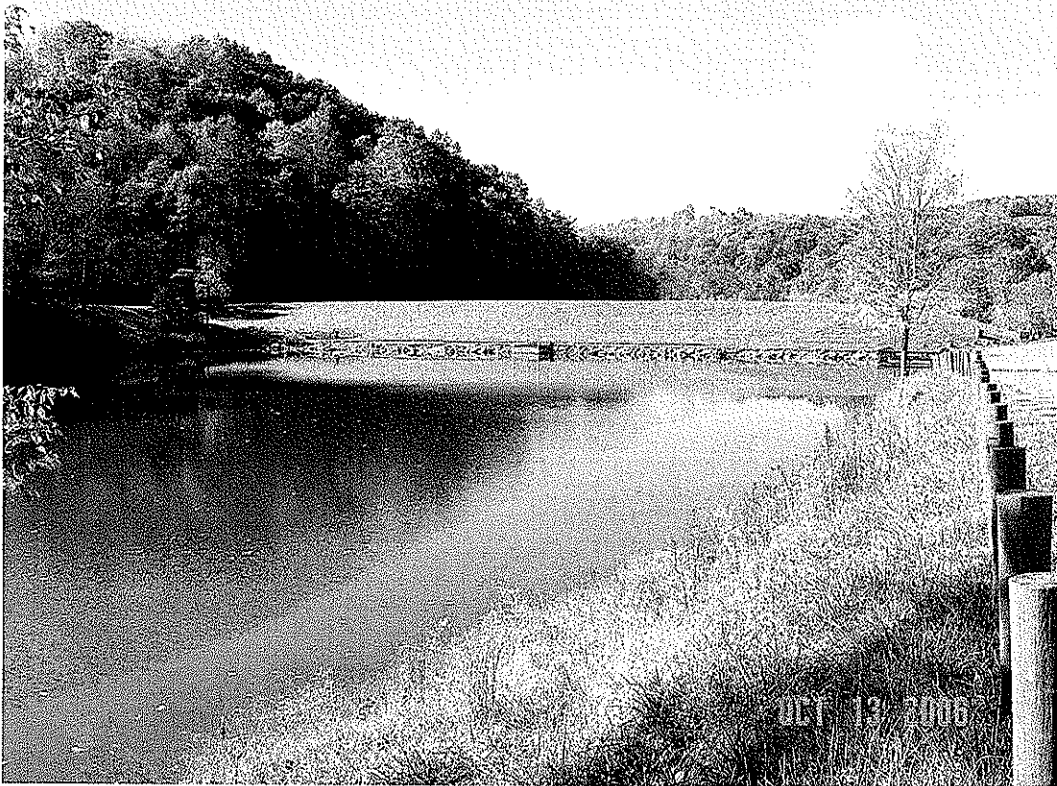
JIMMY LEWIS DAM MODIFICATION, MERCER CO., WV
