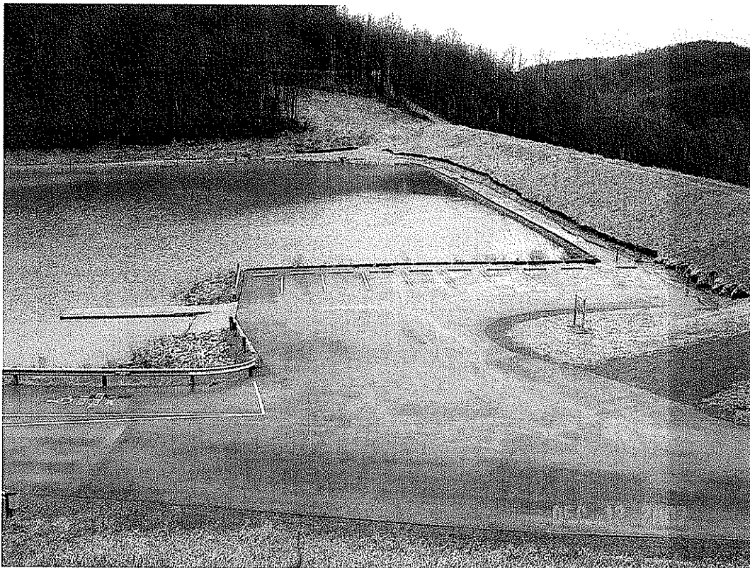
BAILEY DAM MODIFICATION, MONONGALIA CO., WV
