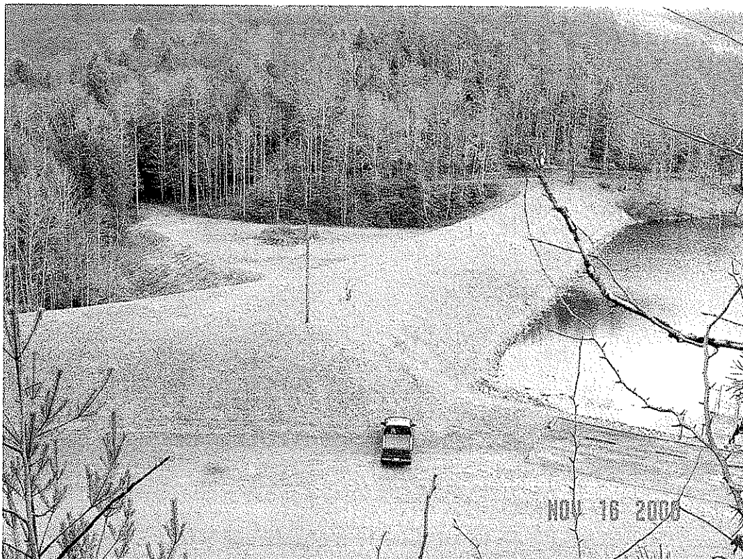
PLUM ORCHARD DAM MODIFICATION, FAYETTE CO., WV
