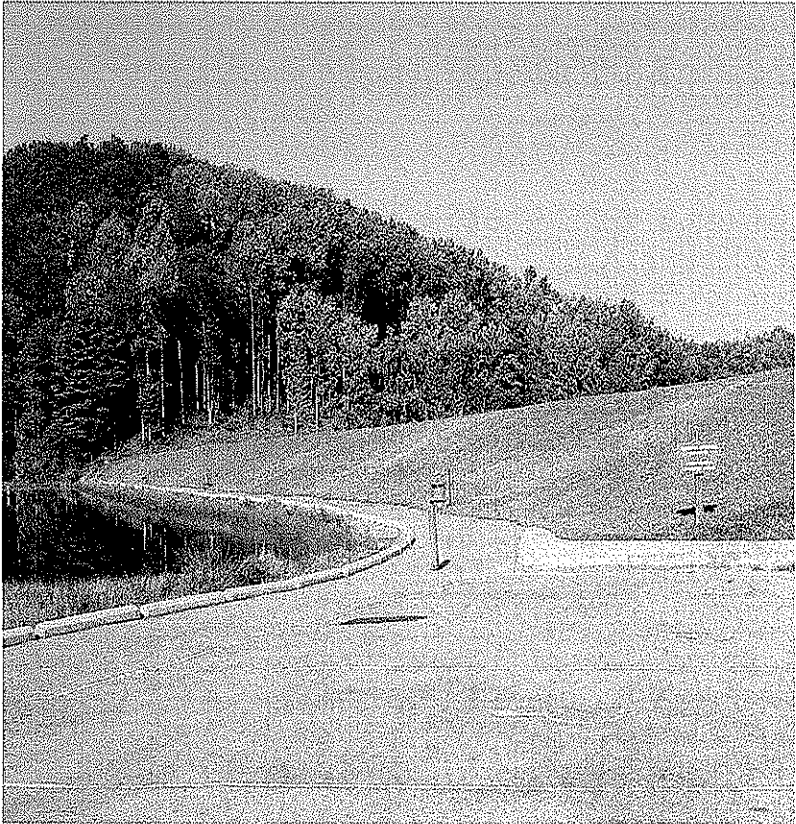
TETER CREEK DAM MODIFICATION, BARBOUR CO., WV
