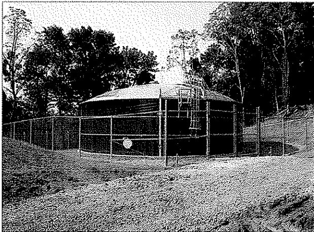
Total Project Cost = $810,000; Completed 2003 New 250,000 Gallon Storage Tank Behind High School
