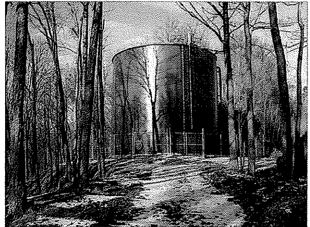
388,000 Gallon Storage Tank Off Route 20 West of Reader
