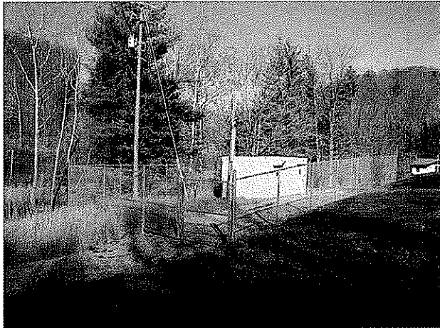
50 GPM Wilsontown Booster Station
