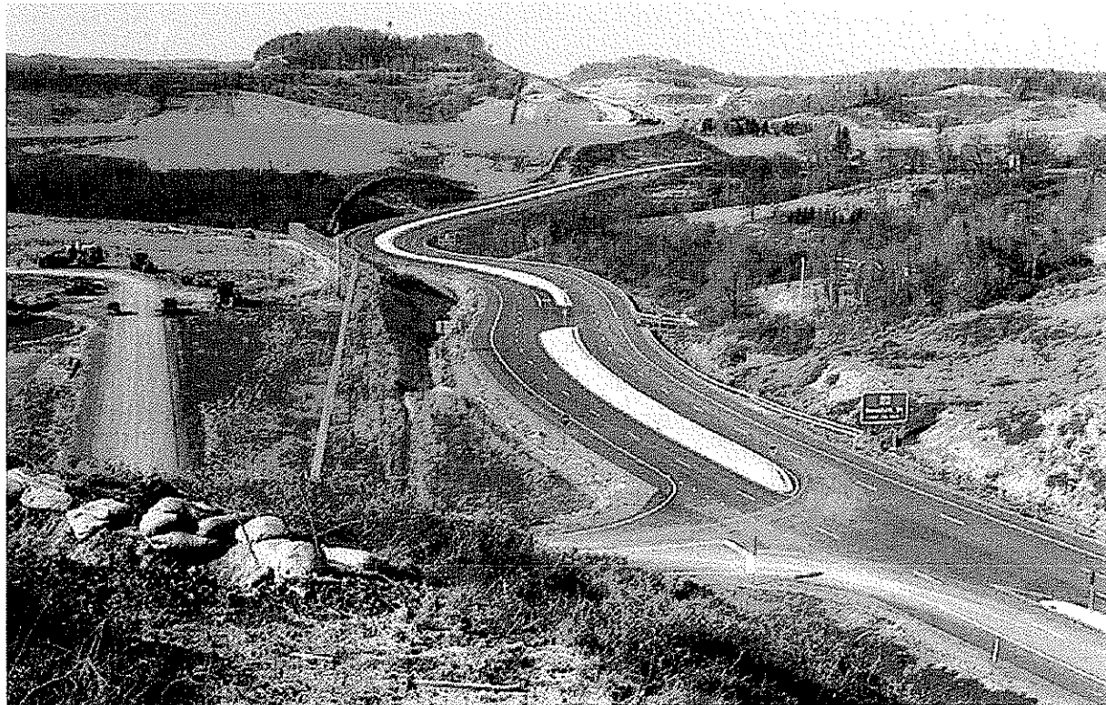
ROUTE 279, NORTH BRIDGEPORT BYPASS - COMPLETED IN 2000
