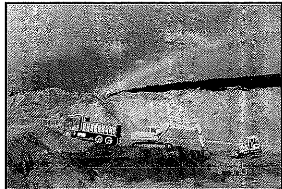
Removal of tailing from floodplain
