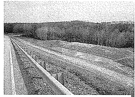
Storm water Pond, Canaan Federal Prison, Scranton, PA
