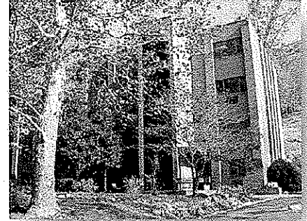
Charleston, West Virginia Office
