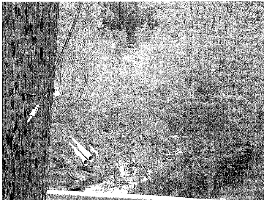
Figure 1—Underdrain Outlet to Grouted Rip-Rap Channel
