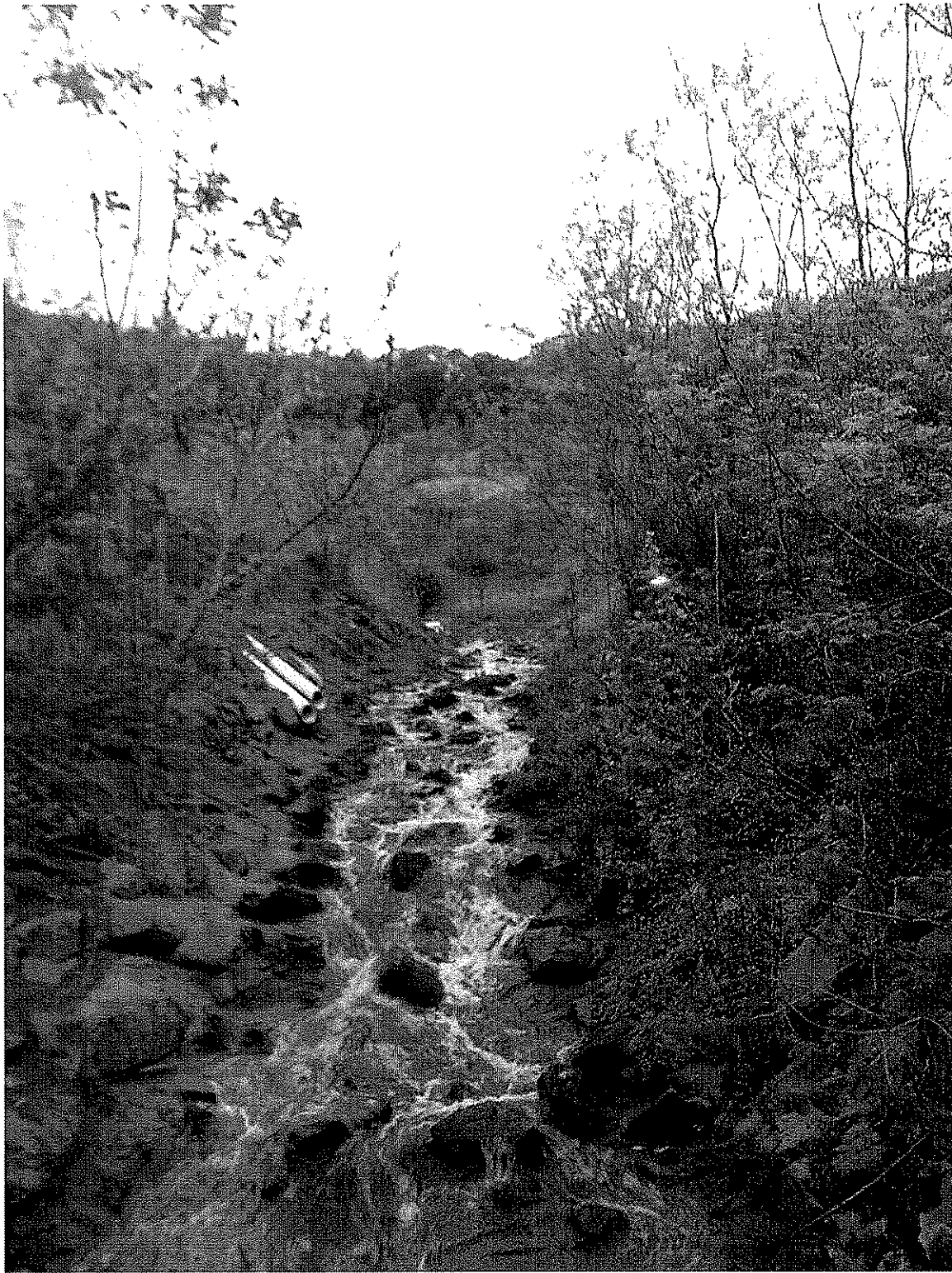
Figure 2—Stabilized Refuse Slopes and Channel with Wet Seal Outlet
