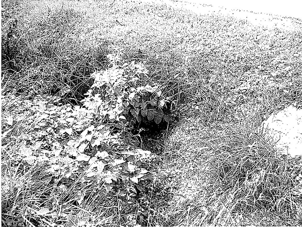
Figure 9—Coal Refuse Clogged Culvert Under County Route 5 on Site 1
