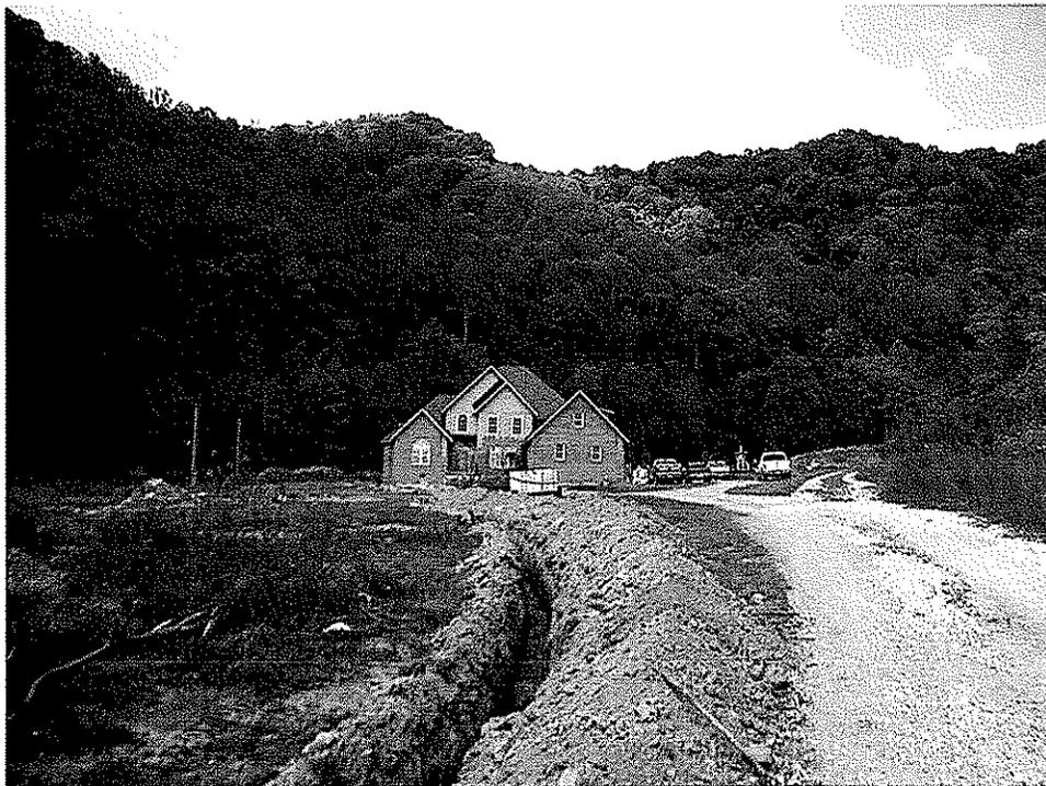
Figure 12—New Home Construction on Site 3. Coal Mine Refuse is Visible in the Water Line Trench
