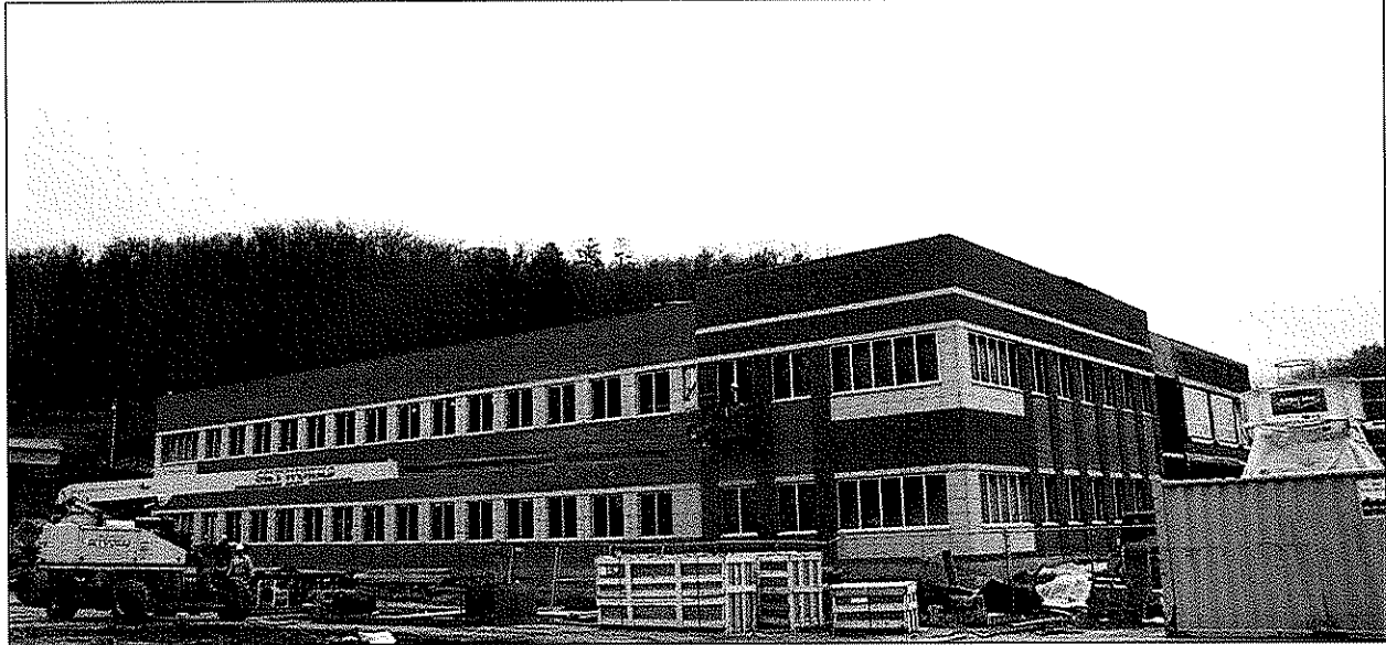
(Currently Under Construction)
