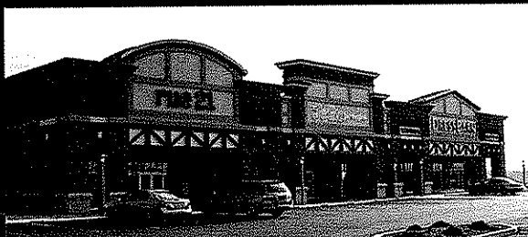
Power Center 'B' Phase 1
