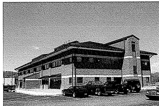
WVDOH D-6 Office Building, Moundsville, WV
