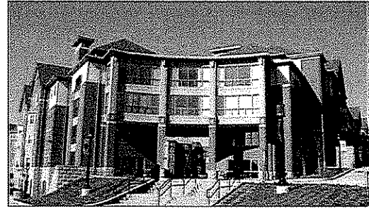
Indiana University of Pennsylvania. The Student Housing Master Plan consisted of 9 buildings to be developed through 4 phases.
