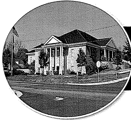
Dayton Municipal Building Dayton, VA
