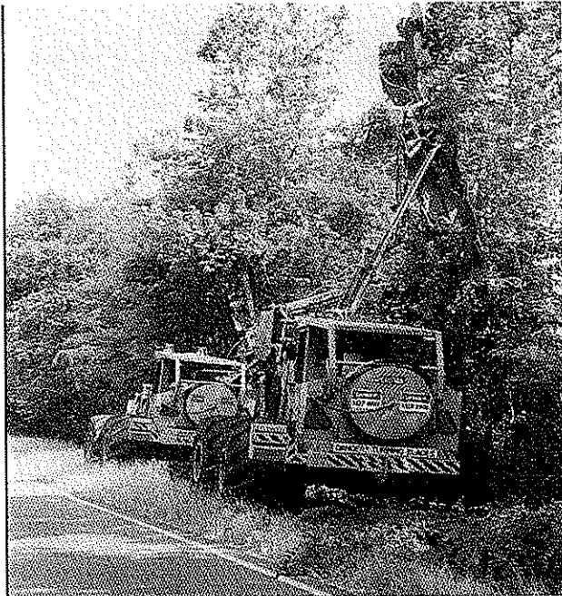
Two Right-of-Way Trimmers in tandem One cutting 18', the other cutting 30'
