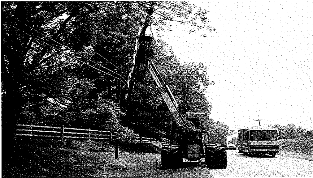
Cutting alongside power lines is no problem
