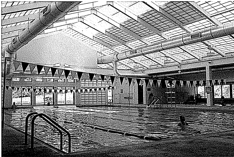
Pool Area w/ Skylite Roof
