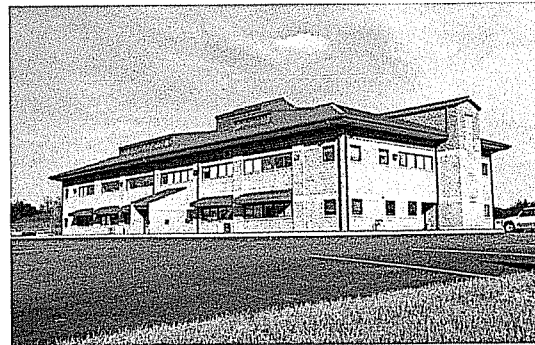
WVDOH D-10 Office Building, Gardner, WV
