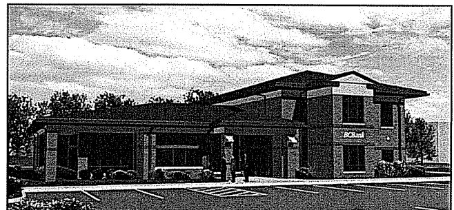
BC Bank Branch Facility Fairmont, WV $2 Million
