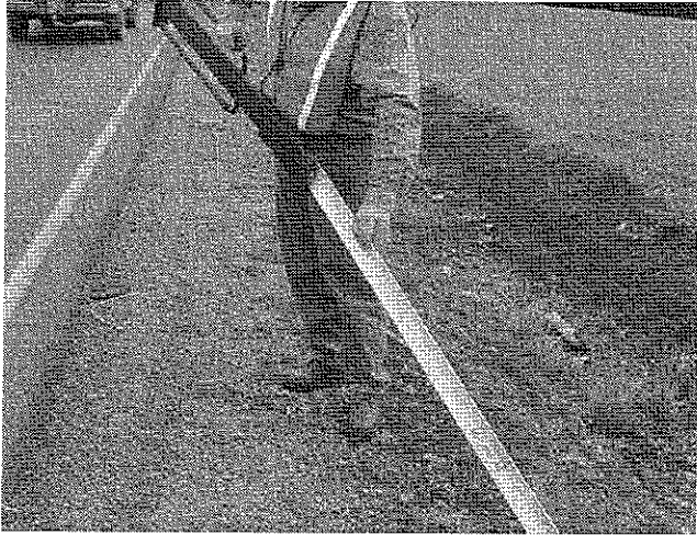
1. Place Delineator Post into Driver
