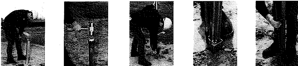
Figure 3: Nex® Sign Support System Installation
