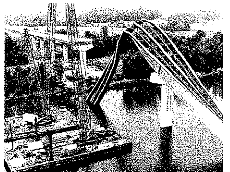
TENNESSEE RIVER BRIDGE THE STATE OF TENNESSEE ENGAGED WJE TO INVESTIGATE THE THREE-SPAN, 1,205-FOOT STATE ROUTE 69 BRIDGE AFTER IT COLLAPSED DURING CONSTRUCTION.
