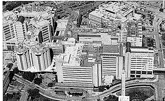
TEXAS MEDICAL CENTER WJE PROVIDED A COMBINATION OF EXTERIOR ENVELOPE CONDITION SURVEYS, REPAIR DESIGNS, AND CONSTRUCTION OBSERVATION SERVICES FOR ELEVEN EXISTING BUILDINGS AT THE M.D. ANDERSON COMPLEX IN HOUSTON'S TEXAS MEDICAL CENTER, AND SERVED AS EXTERIOR ENVELOPE DESIGN CONSULTANT FOR THREE NEW CAMPUS BUILDINGS.
