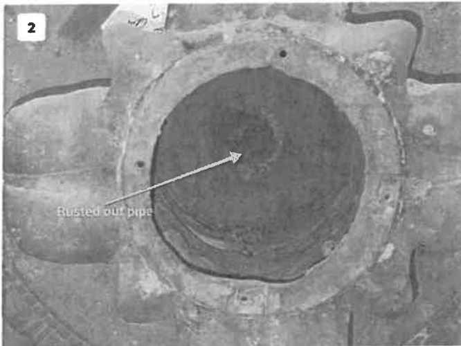
Upper section where main support pipe rusted through
