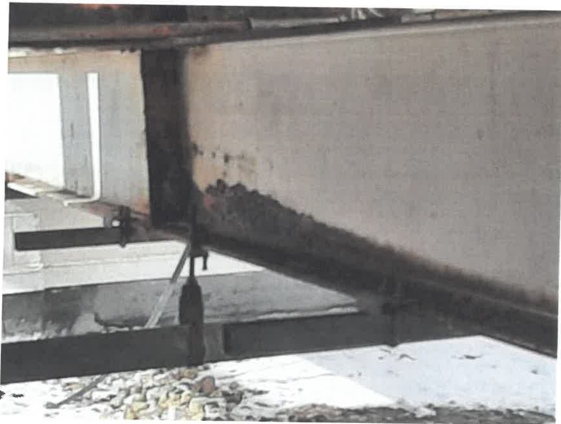
Photo 4. Close-up of Web Deterioration
