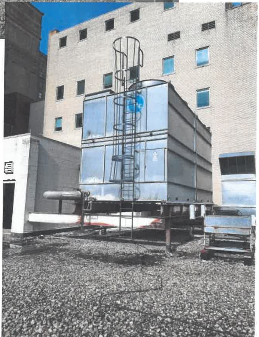
Photo 1. Overall View of Cooling Tower on Roof
