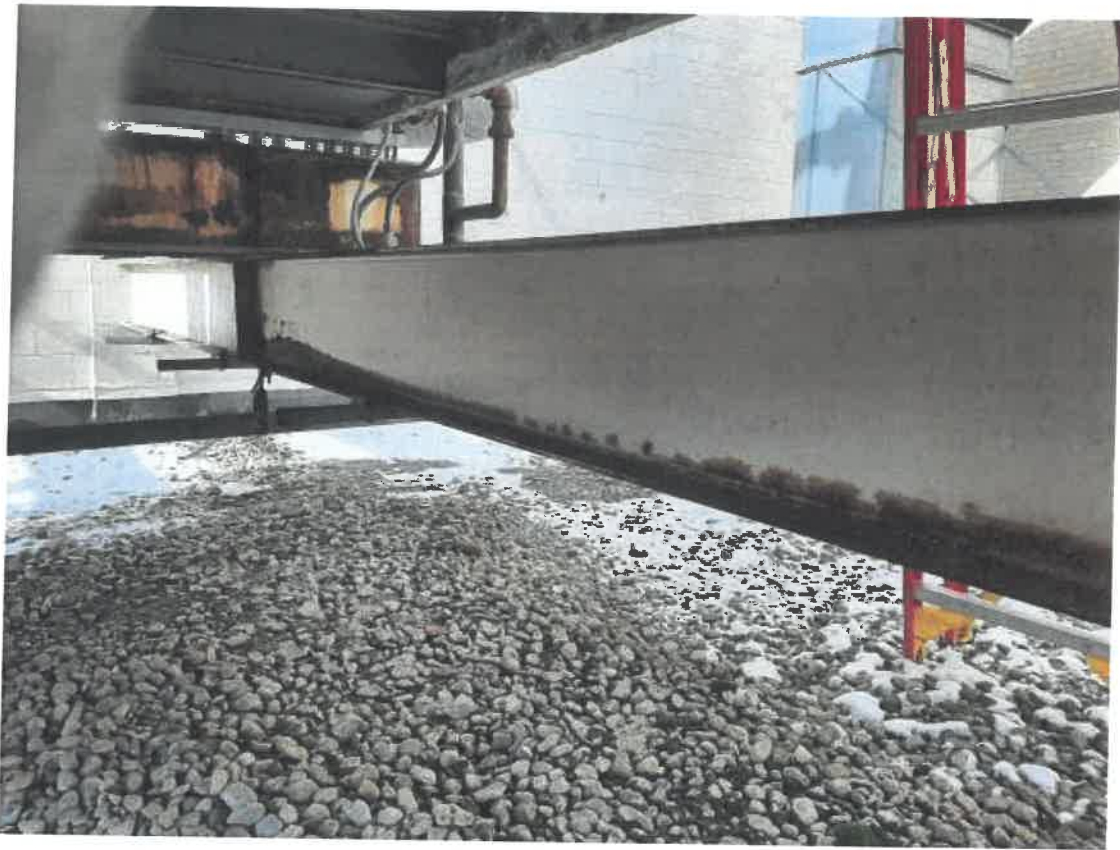
Photo 3. Main Beam with Deterioration on Web
